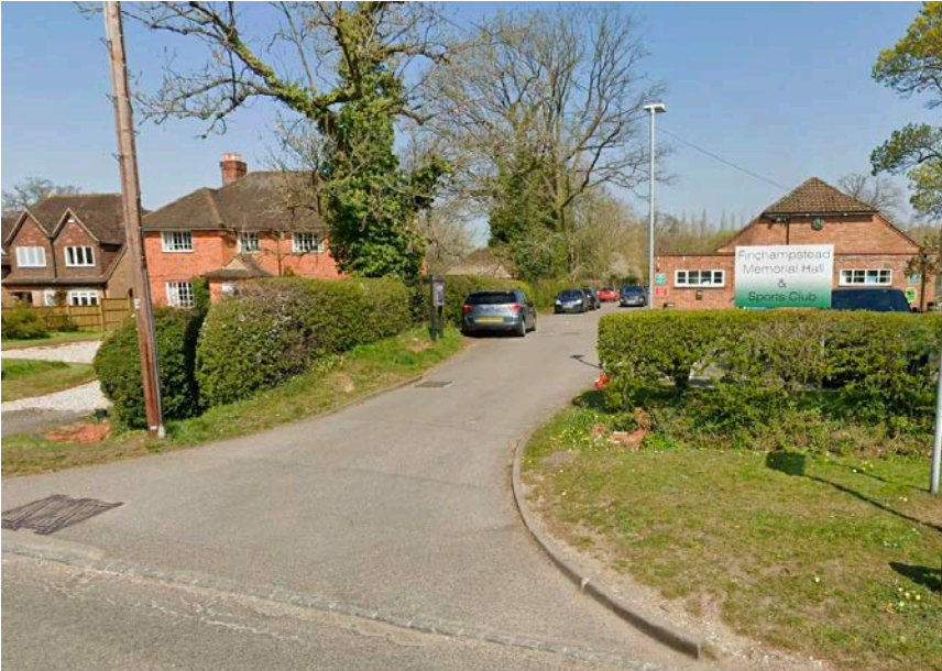
1. The entrance from the B3348.
